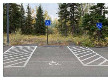
Figure 3.15 Accessible parking space with white parking and white aisle.
