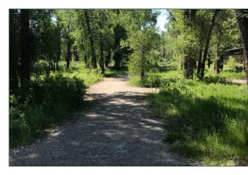
Figure 3.47 Grand Teton National Park, Wyoming, Gros Ventre Campground, six-foot-wide accessible crusher fine aggregate.
