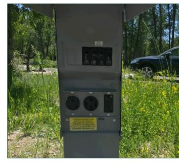
Figure 3.98 Electrical camp site panel with 30amp and 50-amp connections. Consider locking bottom portion of panel to prevent tampering with electrical capacity.
