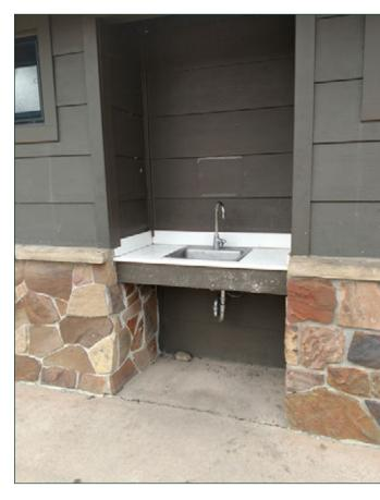
Figure 3.97 The outdoor dish washing sinks at Glacier Basin campground in Rocky Mountain National Park are integrated on the comfort station exteriors and provide a firm and stable surface and knee clearance for accessibility.
