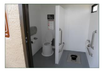
Figure 3.87 Squat toilet adjacent to a standard toilet riser allows users with different preferences to have options.
